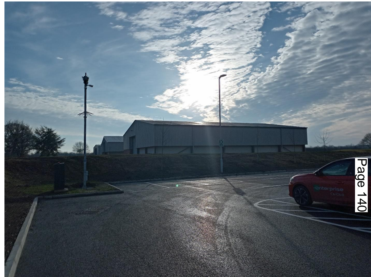
View from neighbouring DPD Car Park
